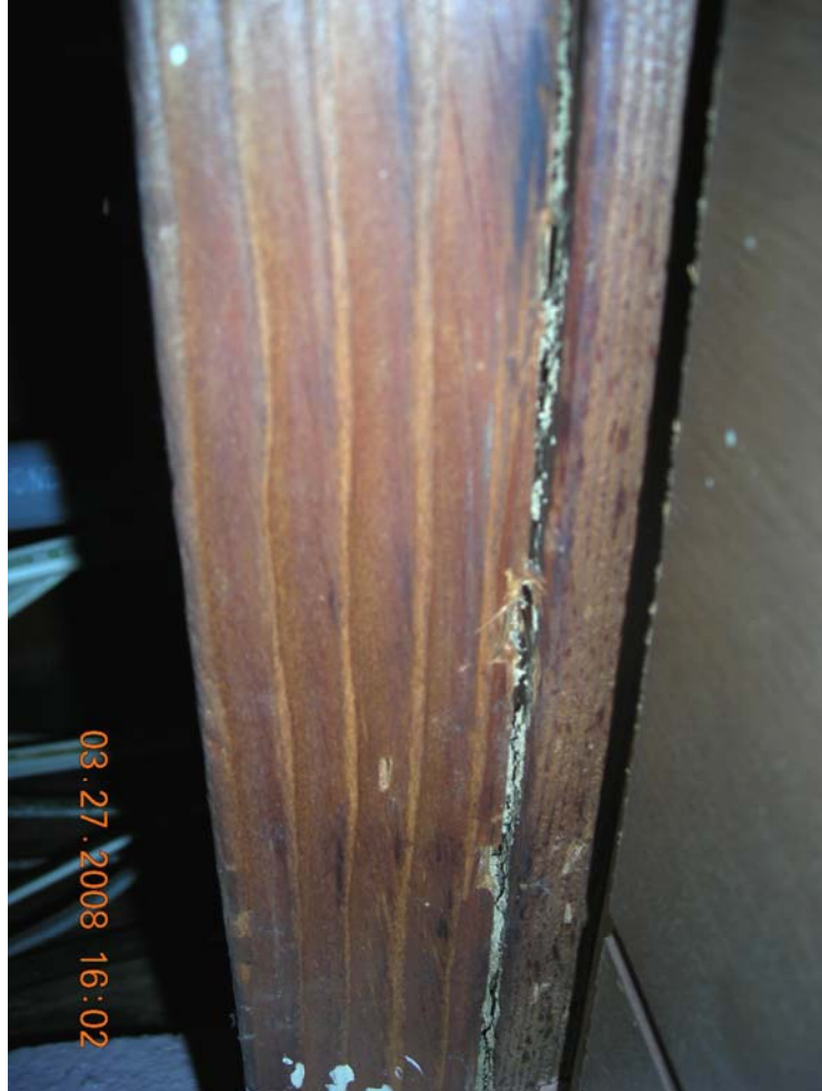
EXHIBIT 7 (Wood Destroying Insect Tubes – Girder)
